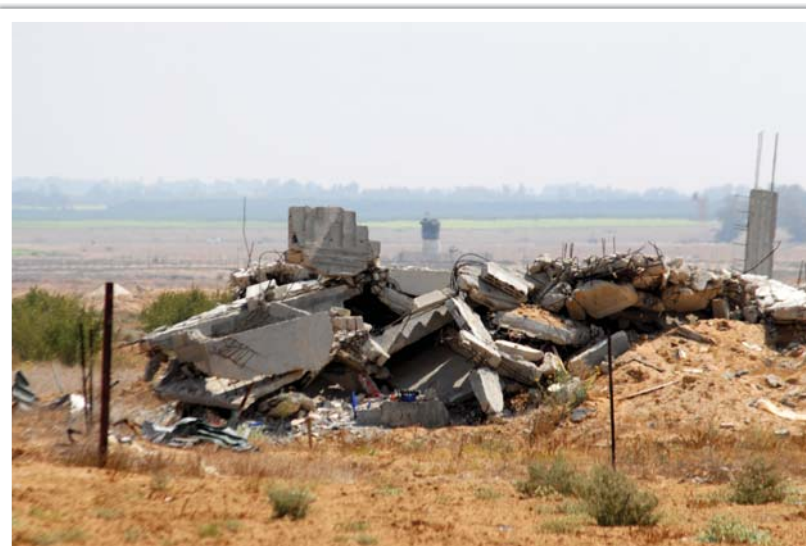
A demolished home in the Fukhkhari area, east of Khan Yunis, very close to the 'no go' area, July 2010
