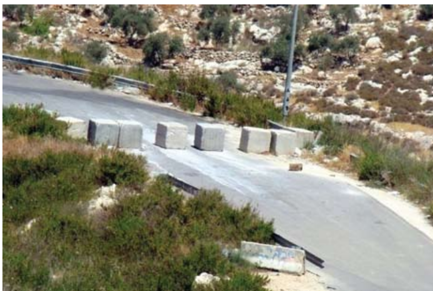
Photo 4: Roadblock in the West Bank
