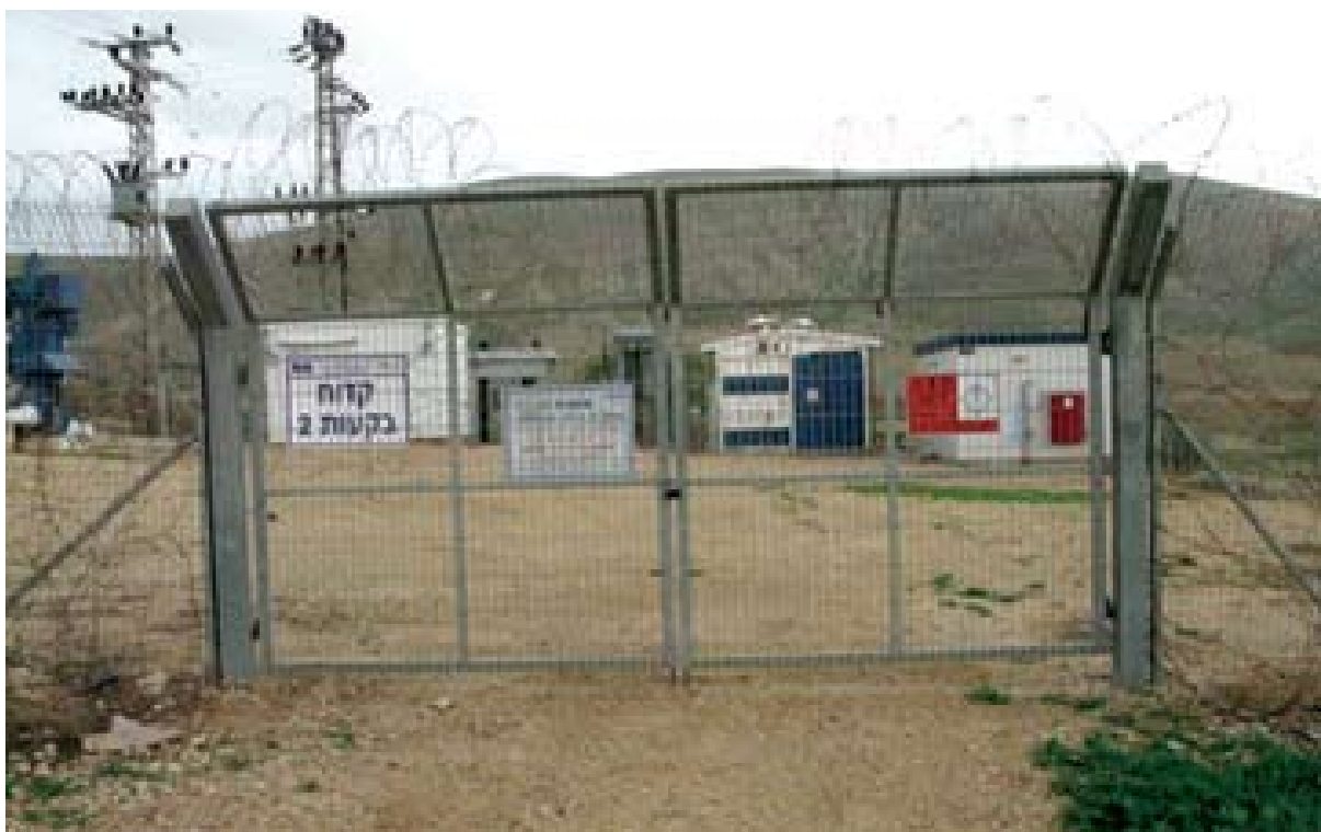
Mekorot water drilling station "Beka'ot 2," next to the Beka'ot settlement, Jordan Valley. (Eyal Hareuveni / B'Tselem, 3 January 2011)
