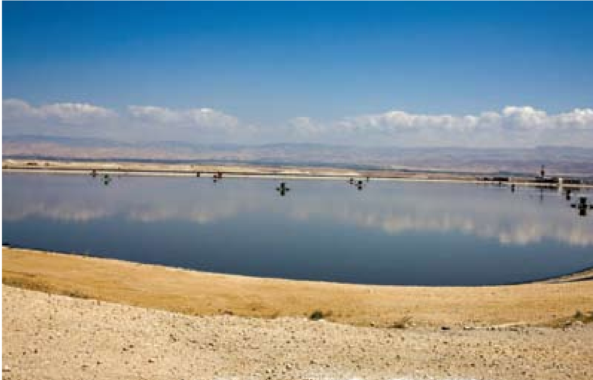
Og wastewater treatment facility, run by Israel, northern Dead Sea area. (Keren Manor / activistills.org, 13 March 2011)
