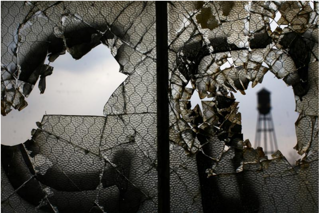
An abandoned manufacturing plant in Detroit, Michigan, April 2011 Eric Thayer / Reuters
